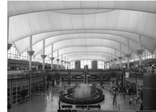
Tensile fiberglass roof in use at Denver International Airport
